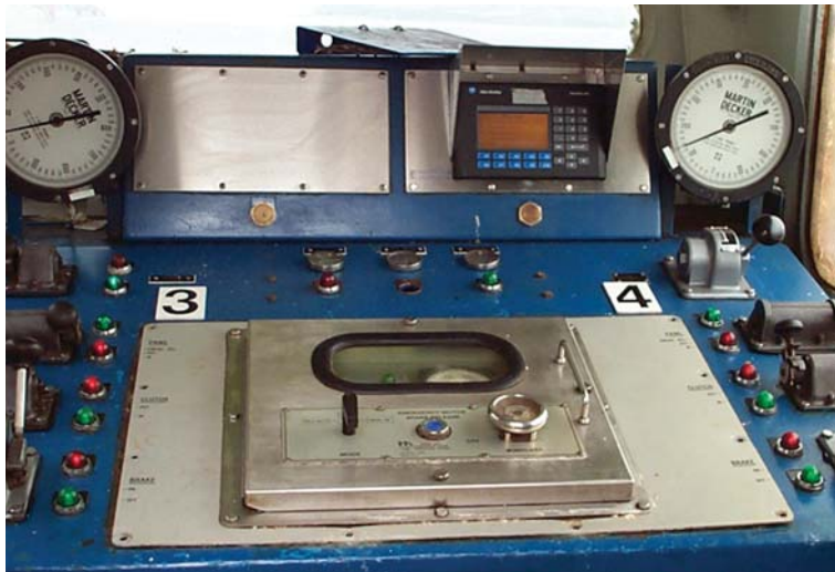
AMS Winch House
