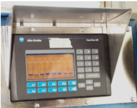
TYPICAL ANCHOR WINCH MONITORING DIGITAL DISPLAYS
